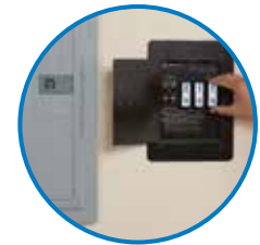
Step 3 Turn on power; green light indicates surge protection has been restored
